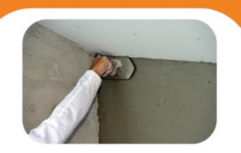
Level the wall with finishing tools; use a corner trowel for corners.
