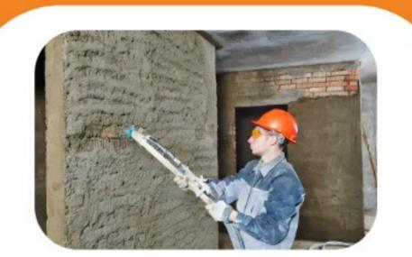
Identify gaps after leveling, respray PrismPlast Spray, and wait for it to set.
