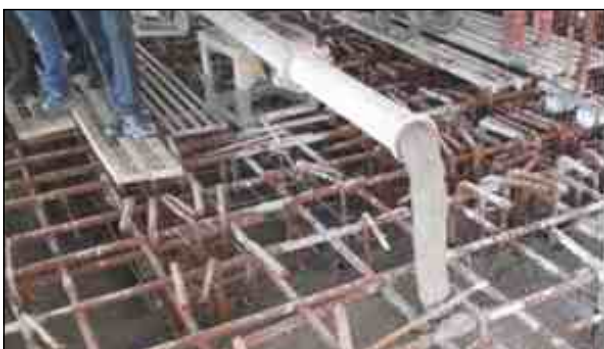
Fig 3 Temperature at pour was well within the specified value of 30°C
