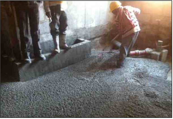
Elitecrete™ being poured in the sunken portion
