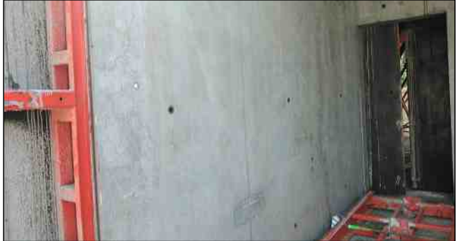
Xpresscrete™ for tunnel form application – good concrete finish eliminates the need of plaster
