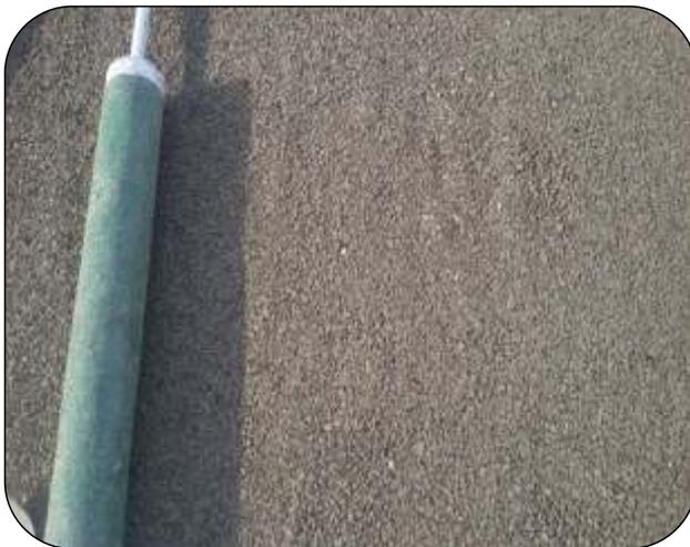
Fig 4 Compaction of *Perviouscrete™* with 65-kg pipe
