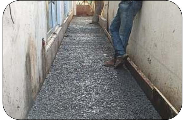
Fig 5 Finished surface of *Perviouscrete™* at Chennai
