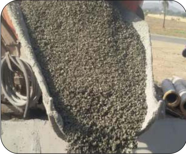
Fig 3 Pouring of *Perviouscrete™*
