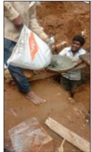
**Fig 5 Portacrete™ is being used for the column starters**
