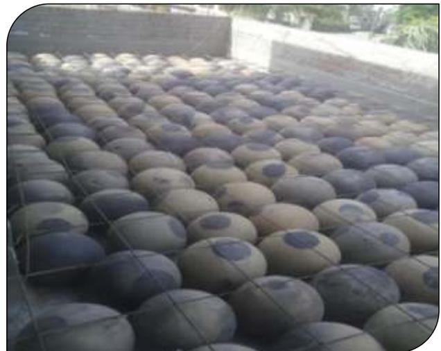
**Fig 2 Ceramic pots placed in rows over the sunken slab**
