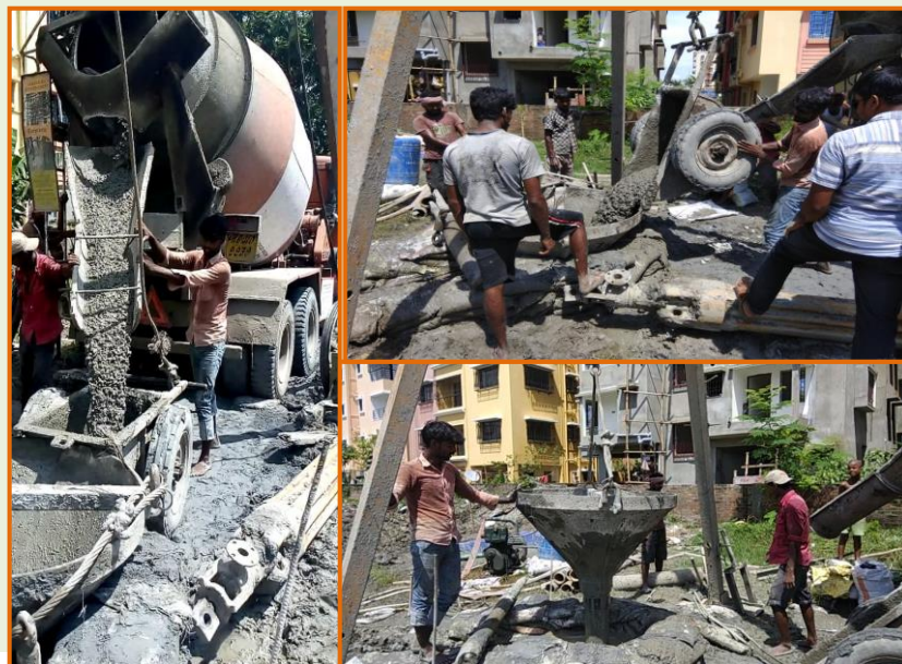
Project site – Pouring going on
