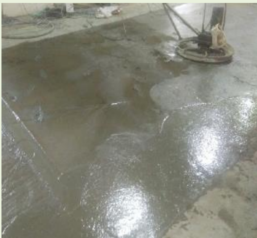
Finishing of concrete with floaters
